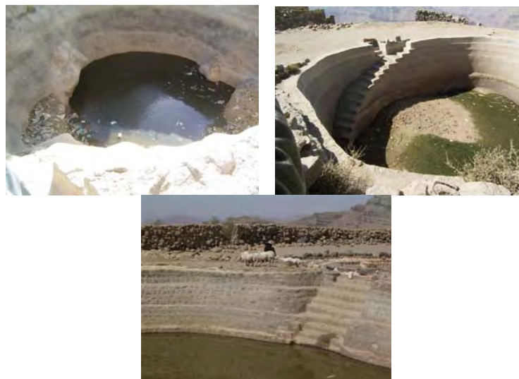
Figure 8: Dirt due to lack of management
