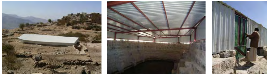
Figure 16: Covered cistern in Al Abr (Khammer)
