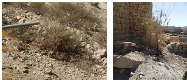
Figure 11: Outlet of the toilet room
