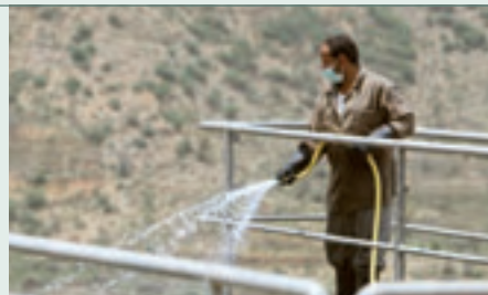
Maintenance of a waste water treatment plant
